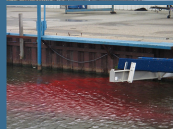
The green dye in this picture confirmed that an illicit discharge was occurring through this storm water outfall along the Clinton River. The dye was put into the sewer cleanout from a facility a half mile away indicating the restroom waste travels directly to the river. The red dye confirmed this marina was discharging sanitary wastewater directly into Lake St. Clair.
