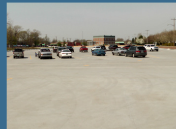
Beneath this parking lot is the Chapaton RTB's 28-million-gallon storage compartment that prevents untreated combined sewage from overflowing into Lake St. Clair. The red brick pump station in the background is capable of pumping up to 700,000 gallons of combined sewage per minute into the facility. Typically, the average E. coli count per 100 milliliters is in the single digits for the discharge from this facility.
